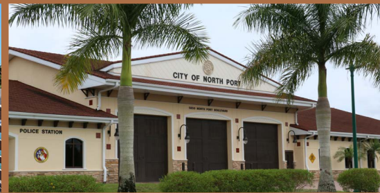
North Port Police Substation, City of North Port
